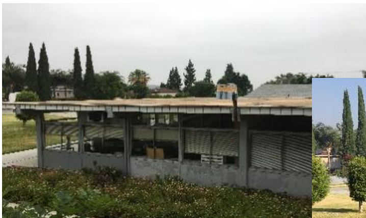
Beginning repair of roof
