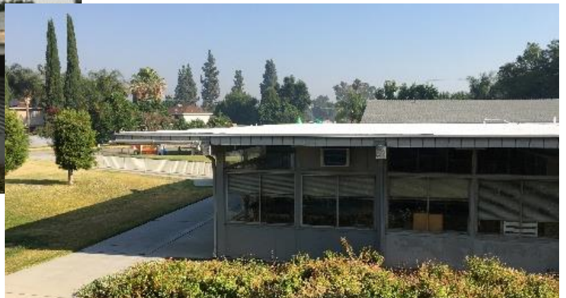
Roof all done!
